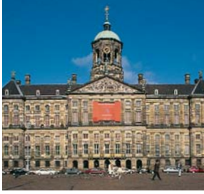
مبنى البلدية mabna al-baladeeya town hall
