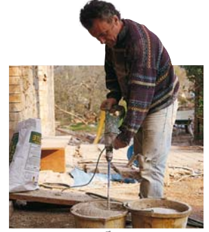
بناء bannaa' construction worker
